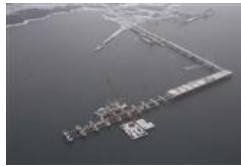
A new deepwater, multi-user iron ore dock under constru...
